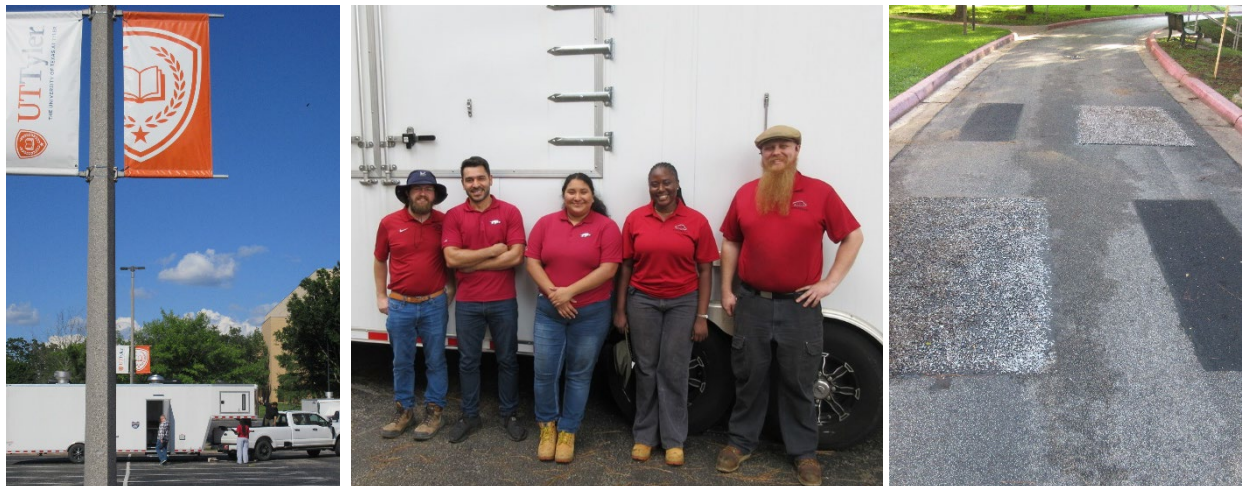
Figure 3 – the trailers arrive at UT-Tyler (left), the TREAT team (center), and the four completed sections (right).
